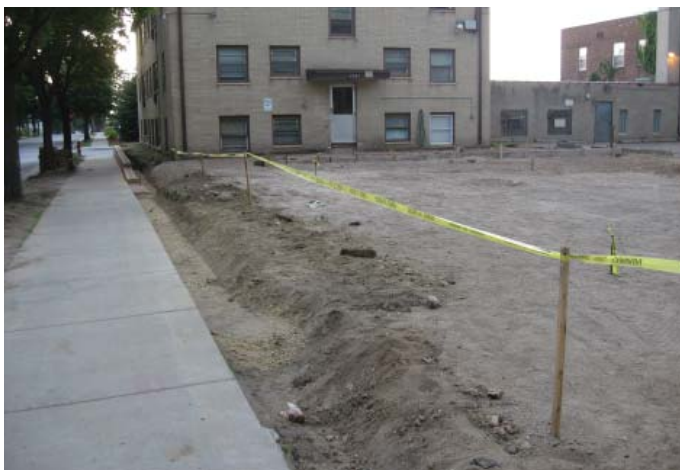
Site just after initial excavation
