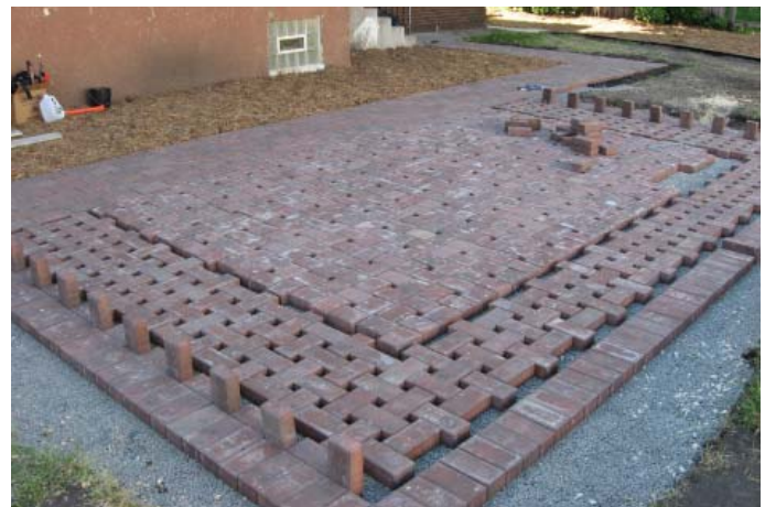
Permeable paver patio installation
