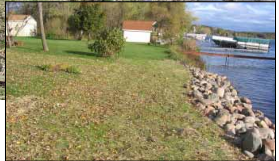
Just after rip-rap installation.
